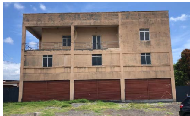
Site 3 before rehabilitation works
